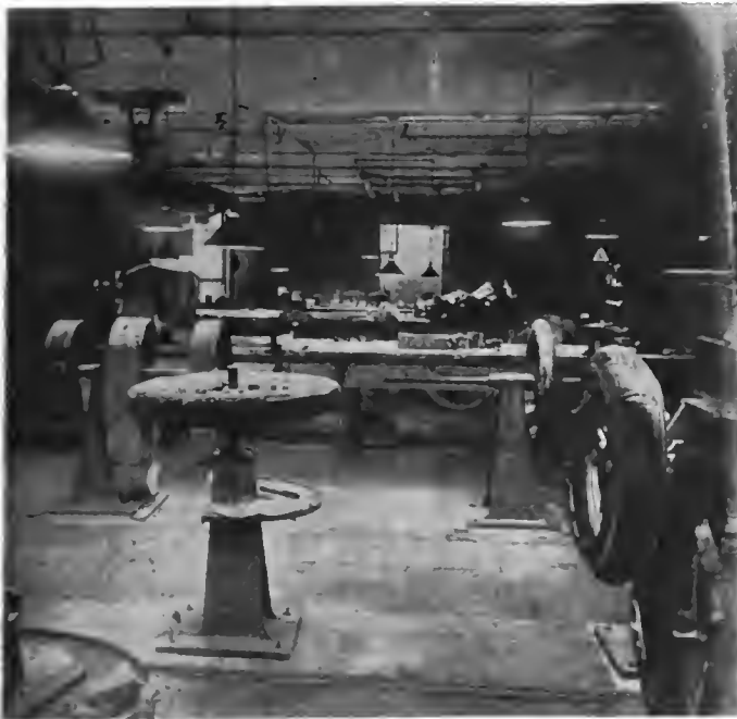
INTERIOR TIRE SHOP EQUIPPED WITH MODERN MACHINERY.
